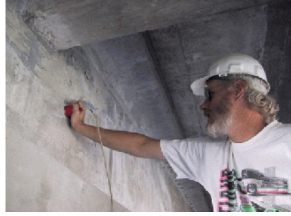
Fig. 6c- UPV Receiver on the West Side of the East Girder
