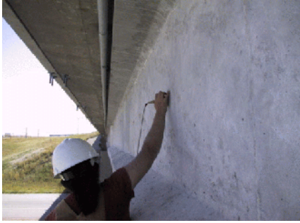
Fig. 6b - UPV Source on the East Side of the East Girder
