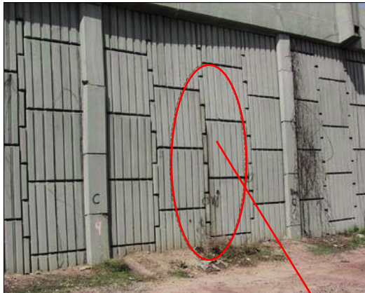
Evidence of water infiltration causing bulging Mechanically Stabilized Earth (MSE) wall correlates to area of high relative mobility.
