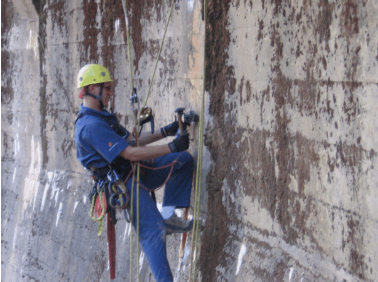
Fig. 2 SASW Testing on Downstream Face of a Dam Using Rope Access
