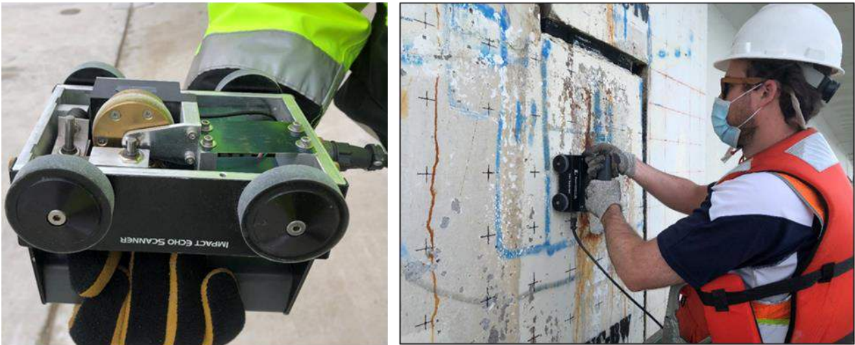
Figure 7: Impact echo scanner with rolling transducer wheel and solenoid impactors (left) and impact echo scanning of girders on vertical lines at 6 in (150 mm) spacing (right)
