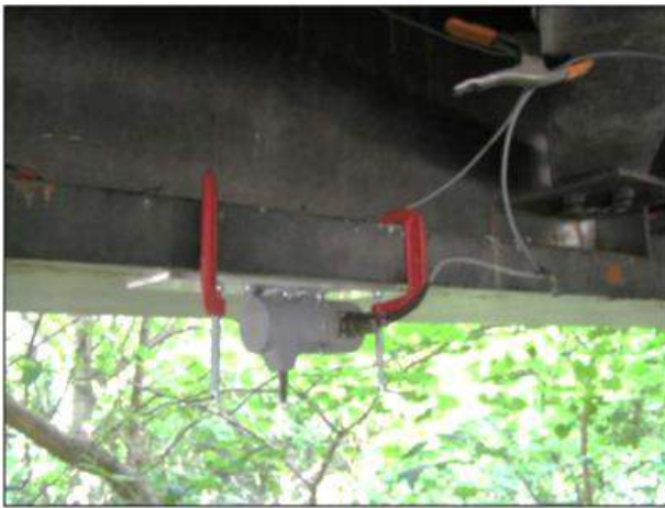
Figure 8. Drexel string potentiometer on Girder 2W3
