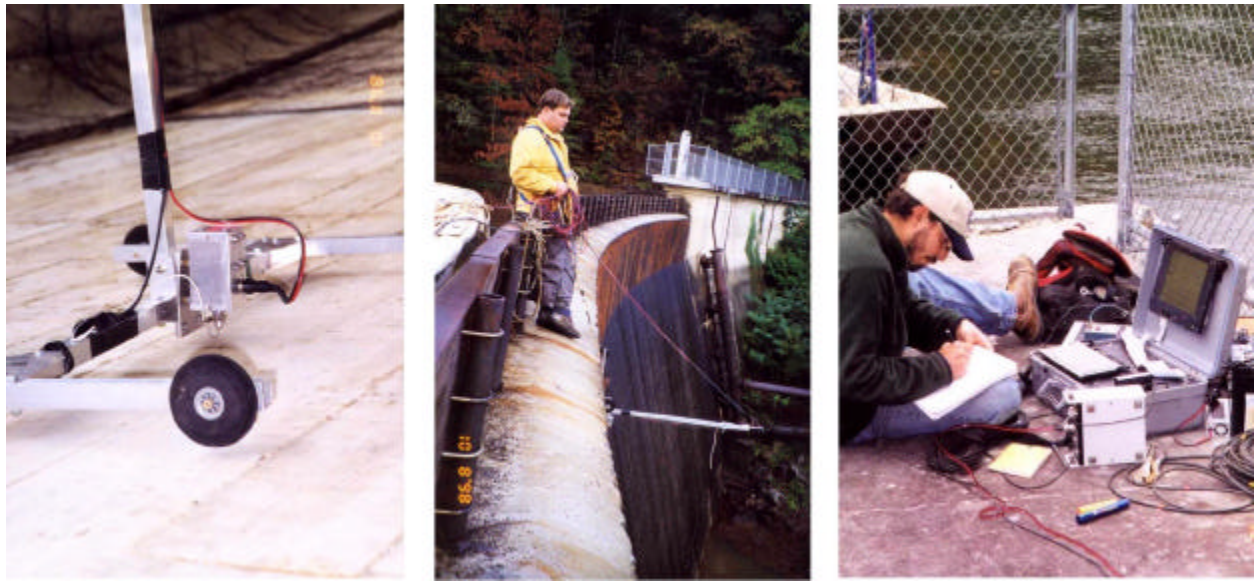
Figure 2. Photographs from October 1998 data acquisition. From left: Closeup of solenoid-actuated sonic impact source; lowering source from top of dam; recording data at station near left abutment. For most stations, the recording unit was in a boat.
