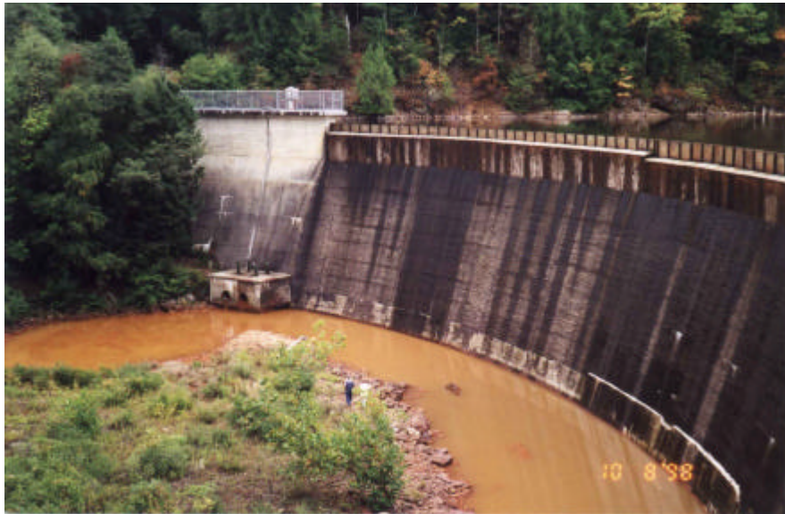
Figure 1. Lake Logan Dam (view from left abutment)
